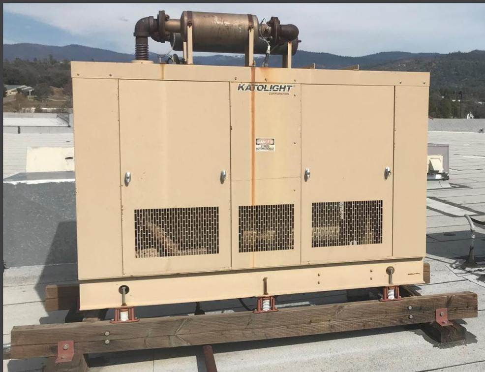
As we discuss in our article "[TOP 6 REASONS WHY YOUR EMERGENCY GENERATOR WILL FAIL TO START](#)", the most common cause of emergency generator failure is battery issues!
